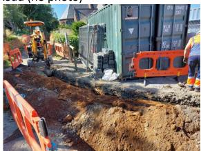
**Building:** Debris removed from under floor and ground compacted (sandstone retained for new entrance to the Cathedral at Derby Road bus stop)
